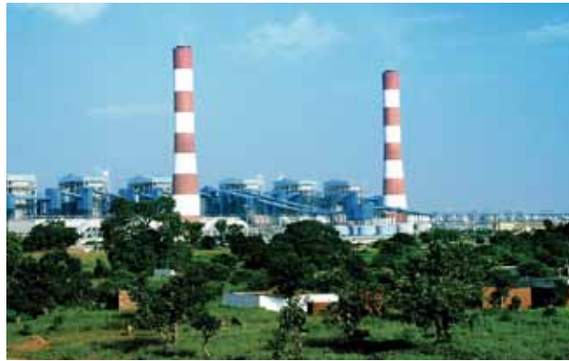
Sasan I Madhya Pradesh 3960MW Ultra mega power project
