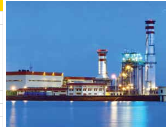
Samalkot I Andhra Pradesh 2400MW Gas-based combined cycle power project
